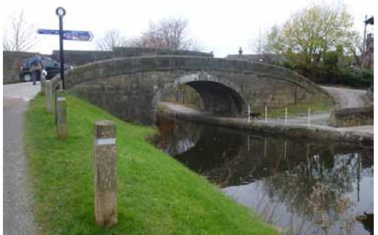
Speed was of the essence as that was where the profits were made. You can probably spot groove marks channelled into the stone by the ropes and metal staples that were introduced to preserve the bridge.
